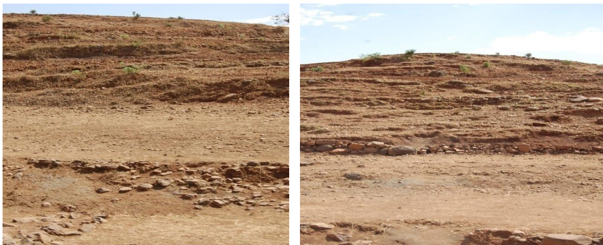
Figure 2: Poorly maintained conservation structures in the study area
